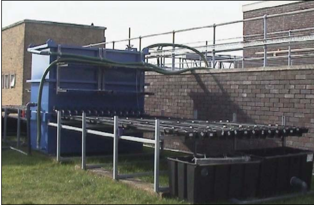
Figure 6. View of the experimental flumes at a London WTW which could be used in chemical dosing trials of BACSAN.
