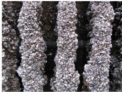
Quagga mussels in the Colorado River, attached to intake towers at Hoover Dam.
